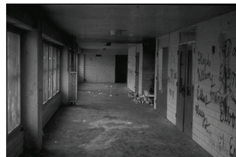
Fig. 2. Image of a vandalised Pruitt-Igoe corridor, Missouri, USA
